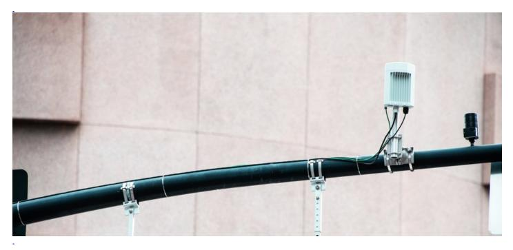
The distributed network infrastructure utilizes Cambium Networks' 60 GHz cnWave™ fixed wireles broadband equipment with Terragraph, a technology developed by Facebook Connectivity.
